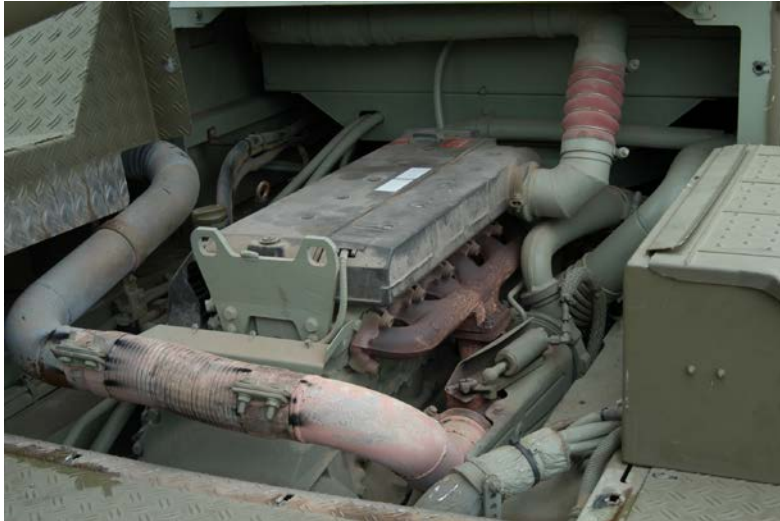
Figure 32A-31: Crane's Engine Compartment
