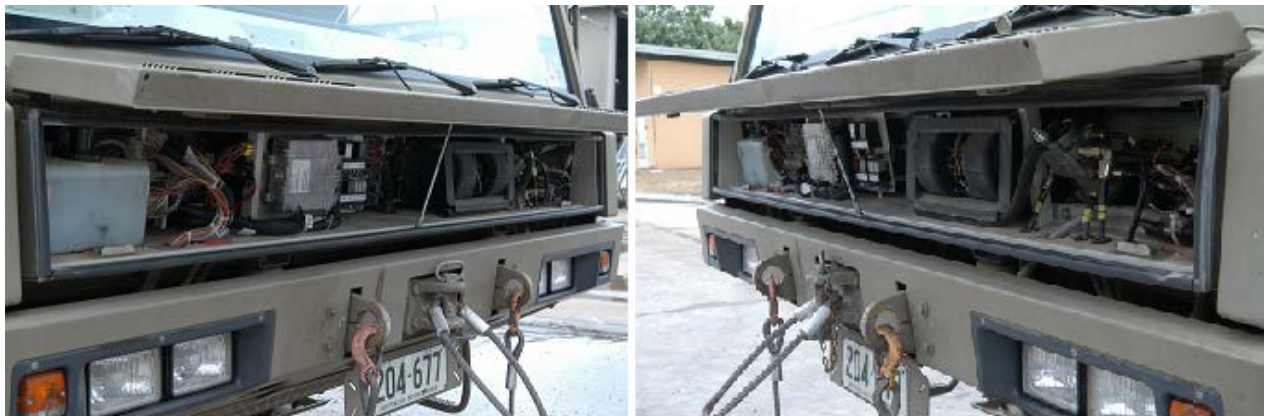
Figure 32A-3: Tadano's Electrical Instrument Fuse Panel
