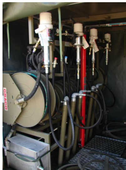
Figure 39–7: Field Lubricating and Servicing Pallet's Hose Reels Internal Side View
