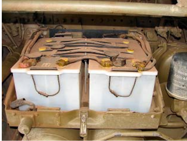
Figure 95-29: Actros Spare Battery Bay
